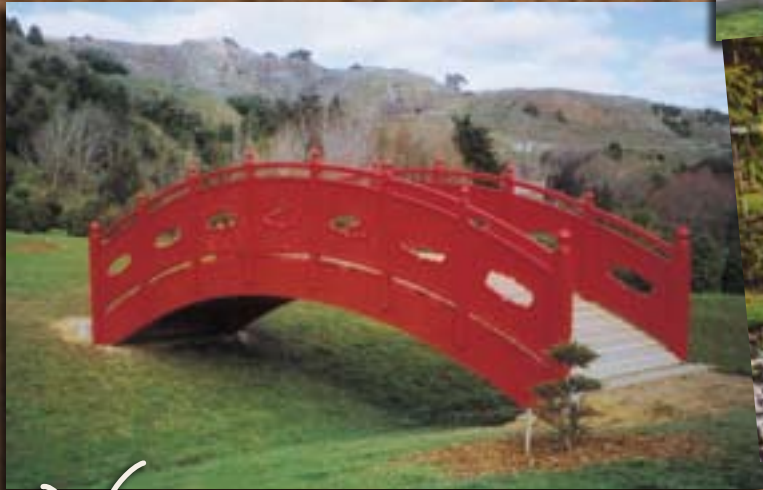
Korean Bridge, Christchurch
